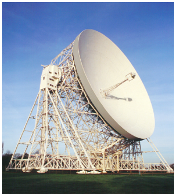
Figure1: The Lovell telescope with its new surface, now aligned to \sim 3\text{mm rms} .
