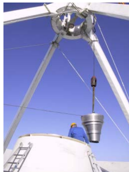
Figure 31: An L-band feedhorn being installed on a MERLIN E-Systems telescope.
