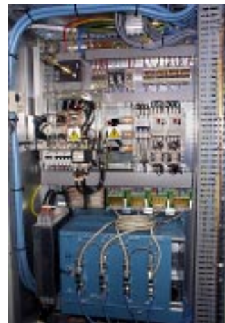
Above: New drive system for the E-systems telescopes.
